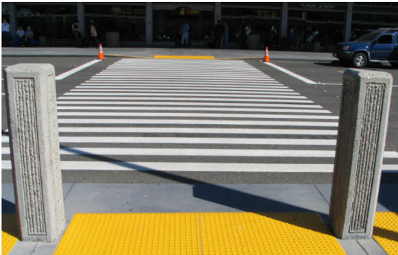
High-quality pedestrian crosswalk markings
