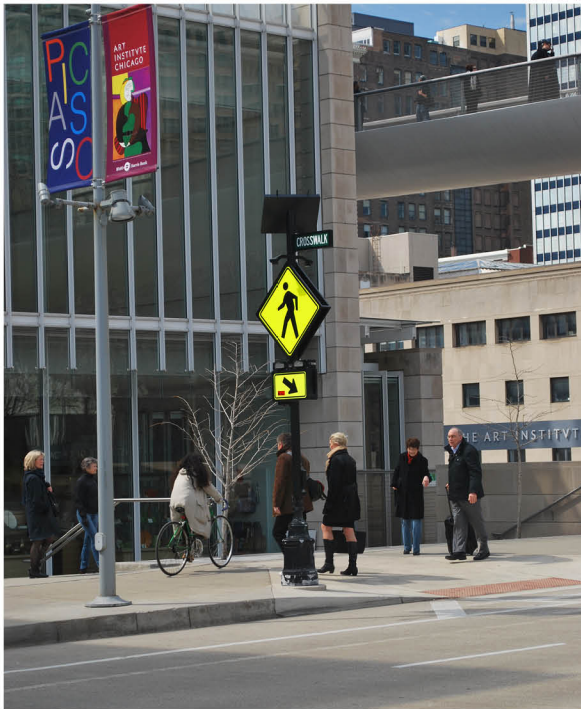
Mid-Block Crossing beacon- solar operated
