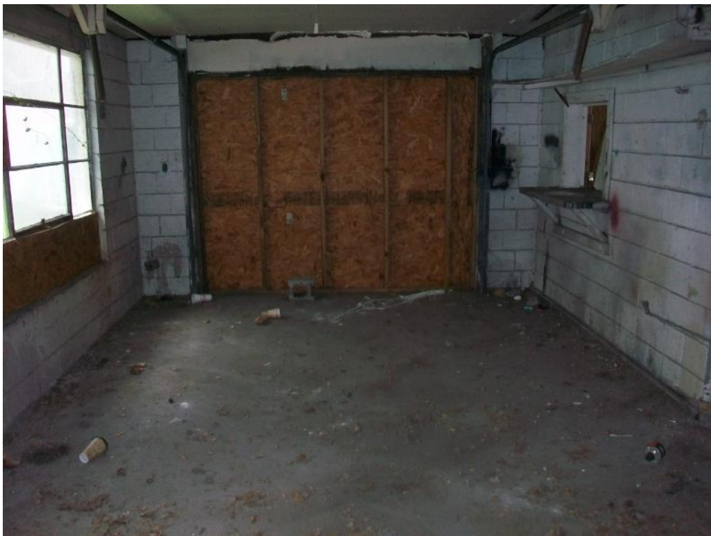
Photograph 7 – View of the garage bay portion of the subject property building.
