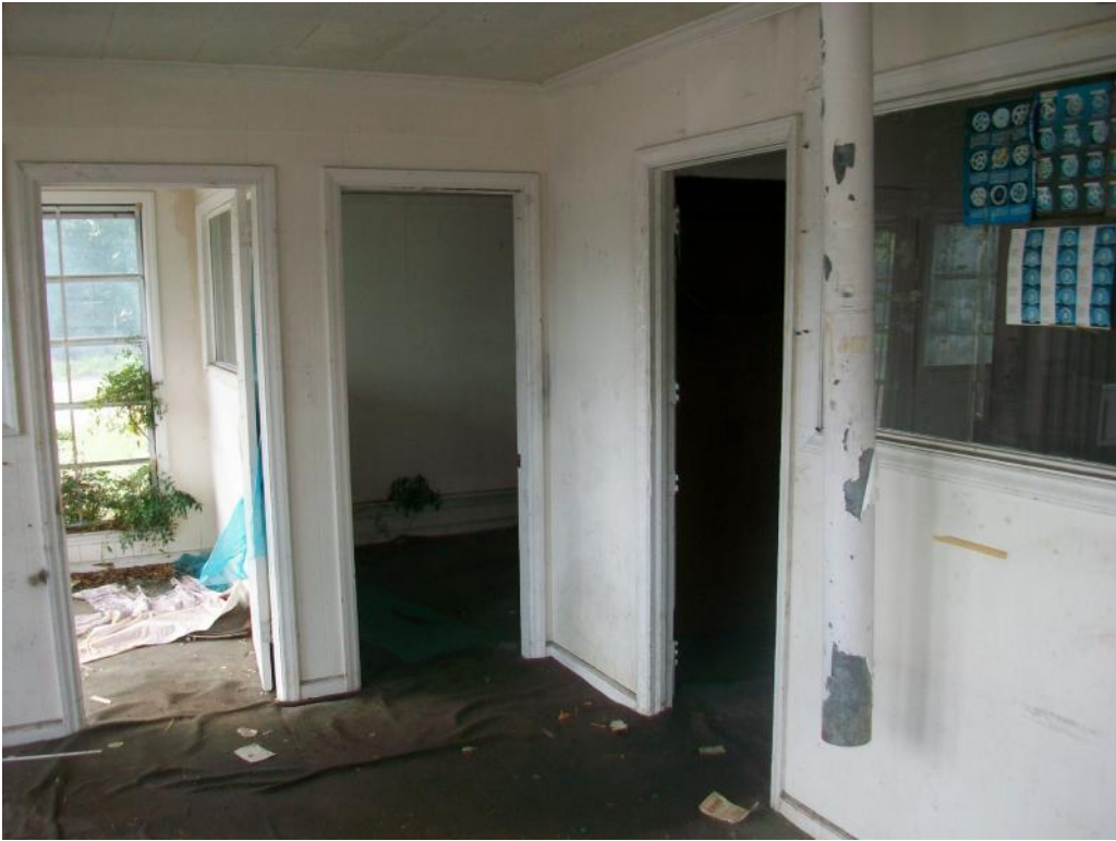
Photograph 9 – Typical view of the office portion of the subject property building.
