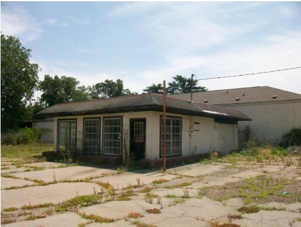
Photograph 2 – View of the subject property building.
