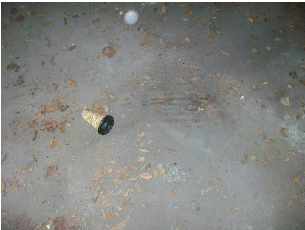
Photograph 8 – View of the floor drain located in the garage bay portion of the subject property building.
