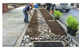
Installation of bioretention bumpout
