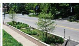
Completed bioretention bumpout
