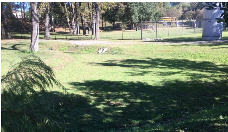
Phase 1 Construction Completed - Earlewood Park bioretention area facing NOMA Dog Park Phase 2 Proposed Construction - Plantings
