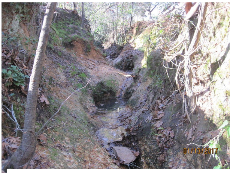
Pre-Construction: Severely eroded and incised tributary to Smith Branch in Earlewood Park before this EPA 319 grant stream bed and bank restoration project.
