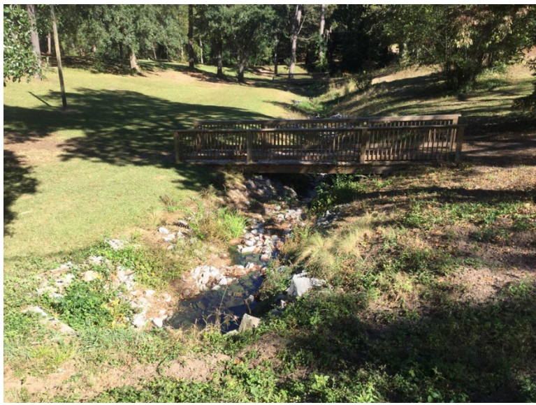
Earlewood Park stream bed and bank restoration area, top facing downstream (November 2021).
