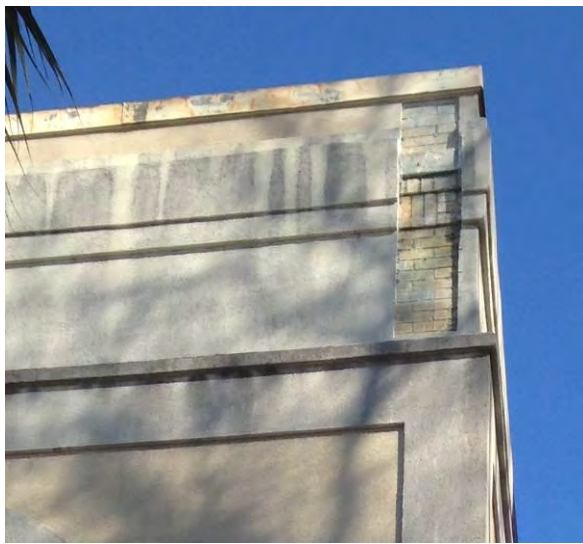
Current images by staff showing exploratory demolition and evidence of intact 1937 facade
