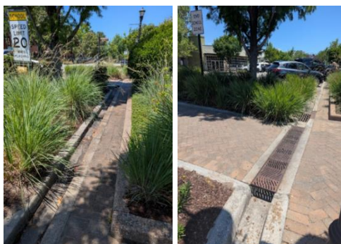
Figure 3: Detached Curb Bump-Outs with grating
