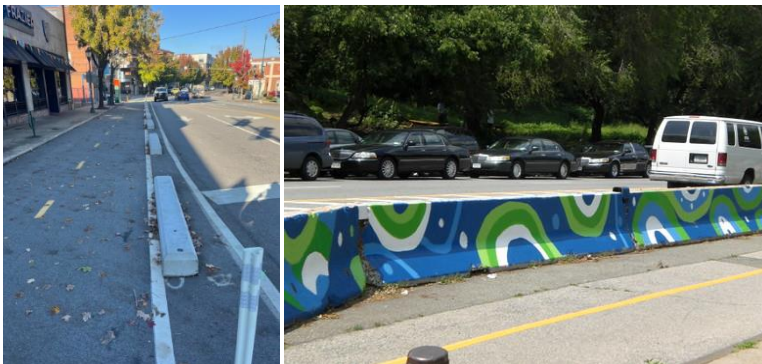
Figure 2: Wheel stop barriers (Left) and Decorative concrete jersey barriers
