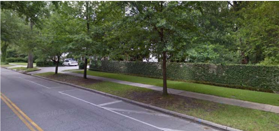
Existing wall, looking south
