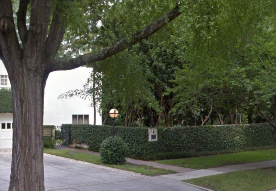
Existing wall, covered with vegetation
