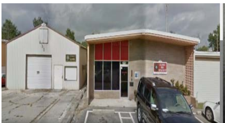
Figure 28. Current Olympia Fire Station
