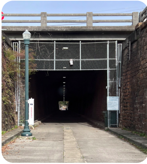
Tunnel Entry South
