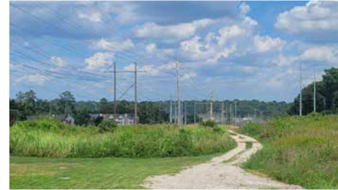
Utility Easement at Skyland Drive
