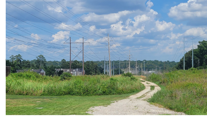
Utility Easement at Skyland Drive
