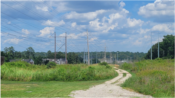
Utility Easement at Skyland Drive
