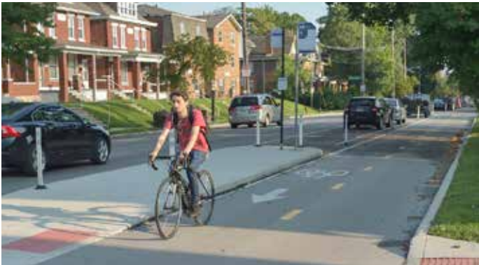
Two-Way Cycle Tracks Bike paths that are physically separated from vehicular (and also often pedestrian) traffic by a barrier or vertical separation (i.e. at sidewalk level) and allow bicycle movement in both directions.
