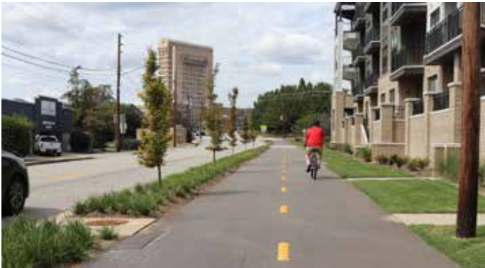
Shared Use Paths A path for pedestrians and cyclists within an existing street right-of-way (next to a road) that is physically separated from vehicular traffic by an open space or a barrier.
