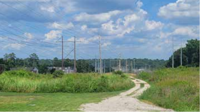
Utility Easement at Skyland Drive
