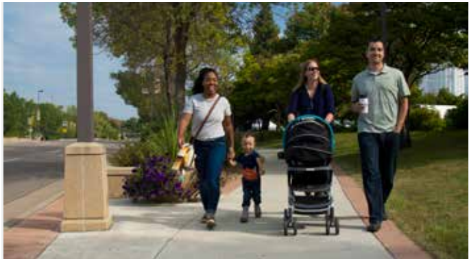
Sidewalks Wide paved path for pedestrians on the side of a road.
