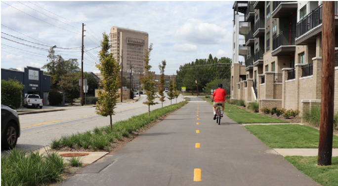
A path for pedestrians and cyclists within an existing street right-of-way (next to a road) that is physically separated from vehicular traffic by an open space or a barrier.
