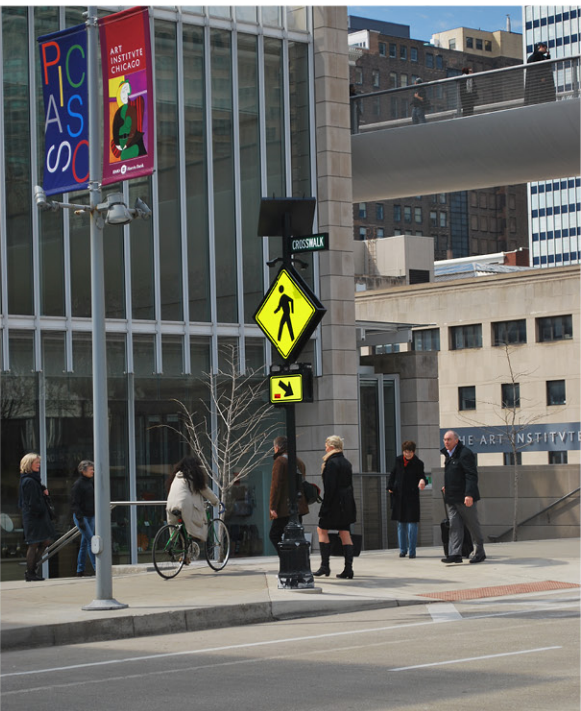
Mid-Block Crossing beacon- solar operated
