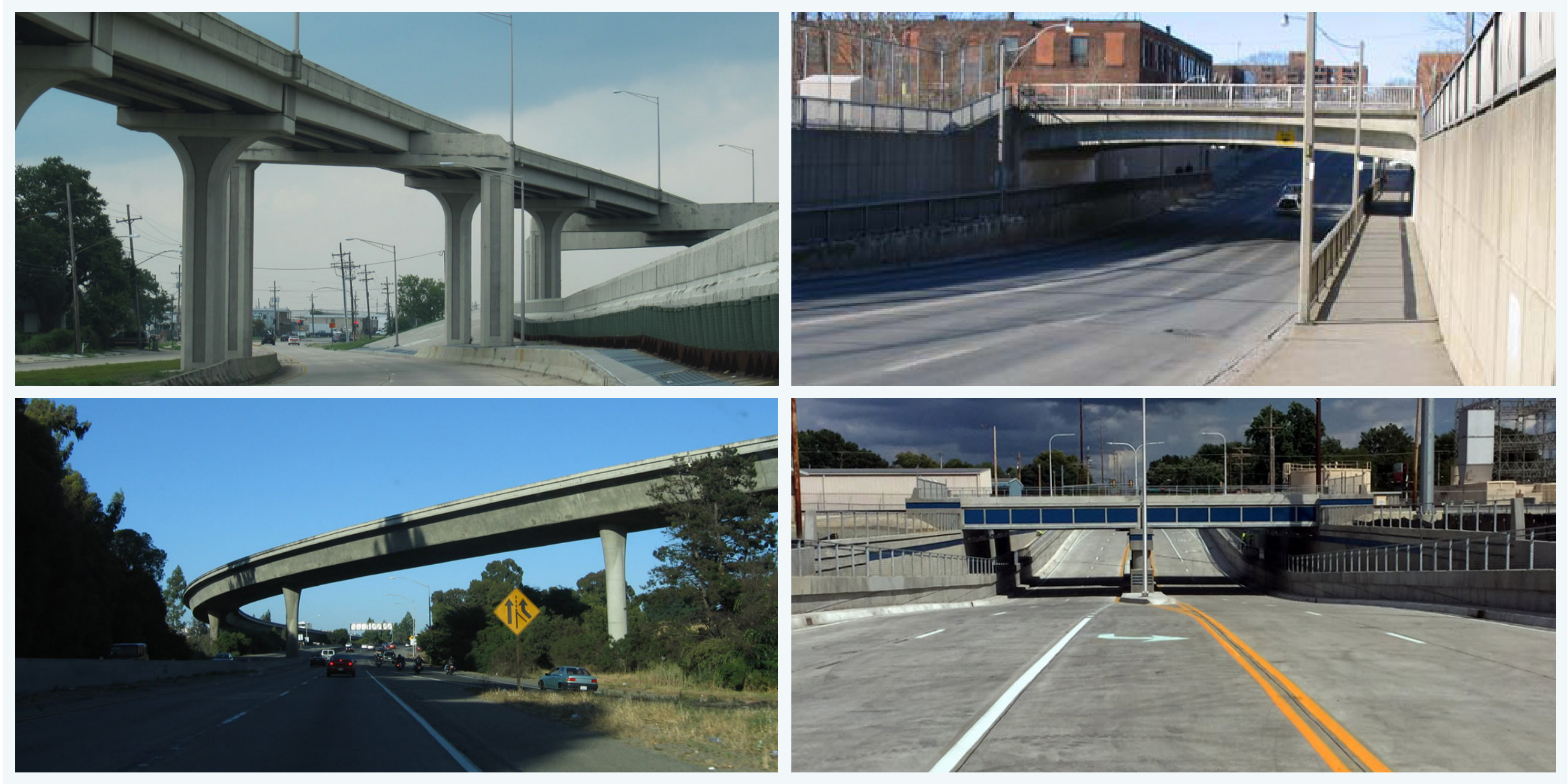
Figure 47: Examples of flyovers and underpasses
